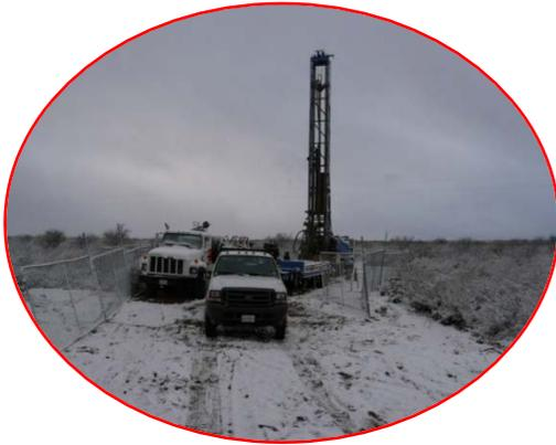
BLM, with the help of the USGS Central Region Drilling, constructed 5 additional monitoring wells in and adjacent to the San Pedro Riparian National Conservation Area. The new monitoring wells will expand the understanding of subsurface geology and will improve the existing monitoring well network within the basin. The knowledge gained from these newly constructed wells will help guide resource management decisions in the future (i.e., locations for recharge projects).
